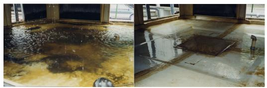
Before and after condition of a Cooling Tower Sump
